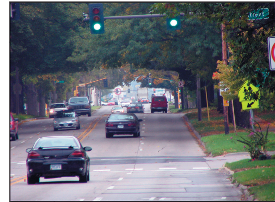
Duff Avenue north of 5th St is one of the most scenic arterial roadways in Ames. The extension of Grand Ave south of Lincoln Way should help reduce expected increases in traffic on Duff Ave and Lincoln Way.
