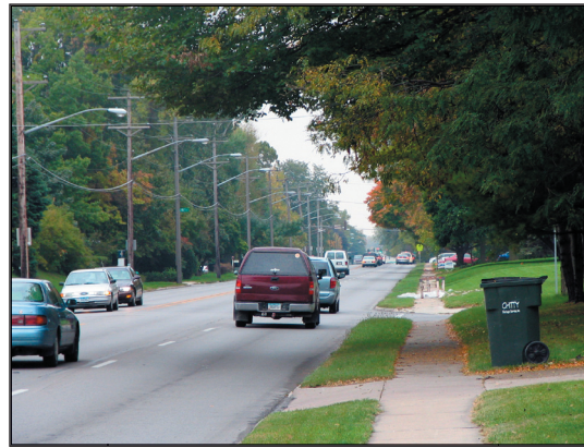
Grand Avenue from 13th St to 20th Street currently does not have left turn lanes. This plan recommends left turn lanes be constructed at 20th St and 13th St.
