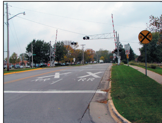
The UPRR crossing on North Dakota Ave was included as a project in the latter years of this plan. It will reduce delays and improve safety on this important arterial street.
